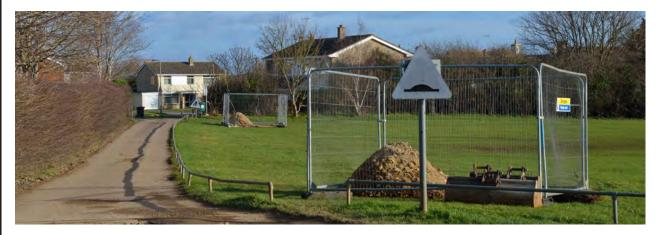
You may have seen some temporary excavations in the field in mid-January (above); test holes were dug to establish ground conditions ahead of construction, and they were refilled when the survey was completed.
